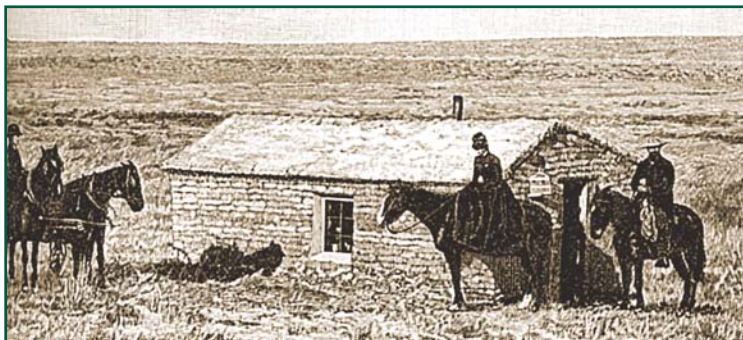
Some homesteaders constructed their houses with sod bricks. They battled nature, illness and loneliness daily. Settlers often lived far apart from their neighbors and might go for months without seeing another family.
